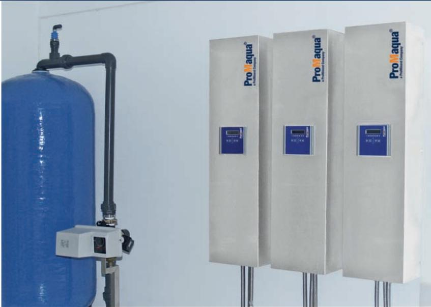
The Dulcoclean® UF eco is a compact ultrafiltration system in the lower capacity range ready for connection.
