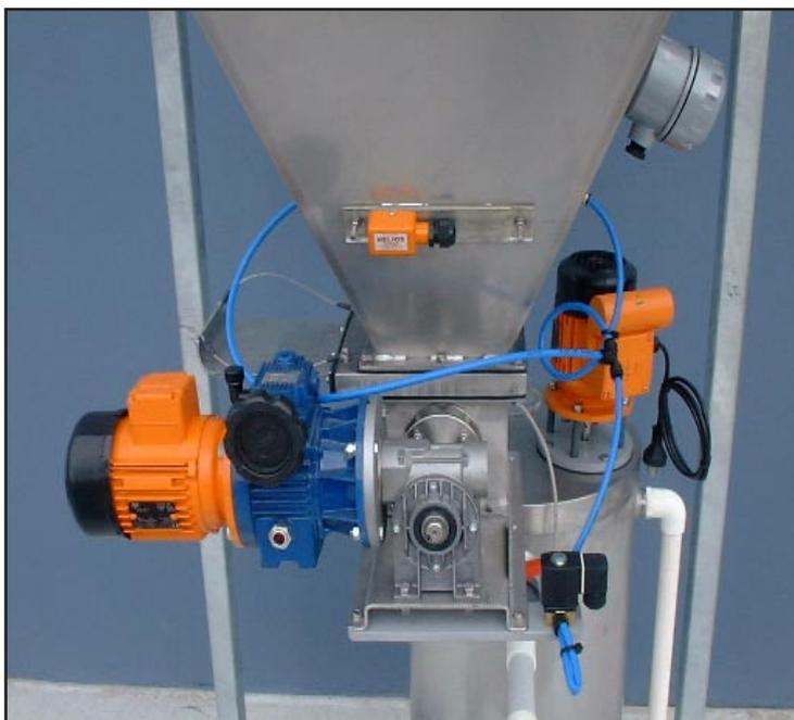
Lime from the storage hopper is metered into the solution tank by the dry chemical feeder. The feeder can be isolated from the storage hopper via a slide gate, allowing the feeder to be serviced without emptying the hopper.
